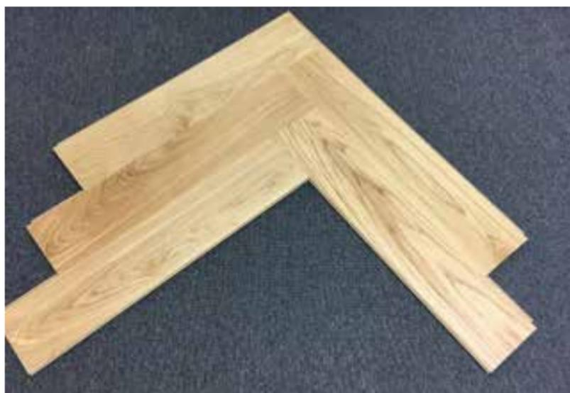
Cut the triangle according to the line indicated below. Depending on the kind of saw that you use, it may be useful to dismantle the triangle before sawing. The excess (below the line) is to be saved.
