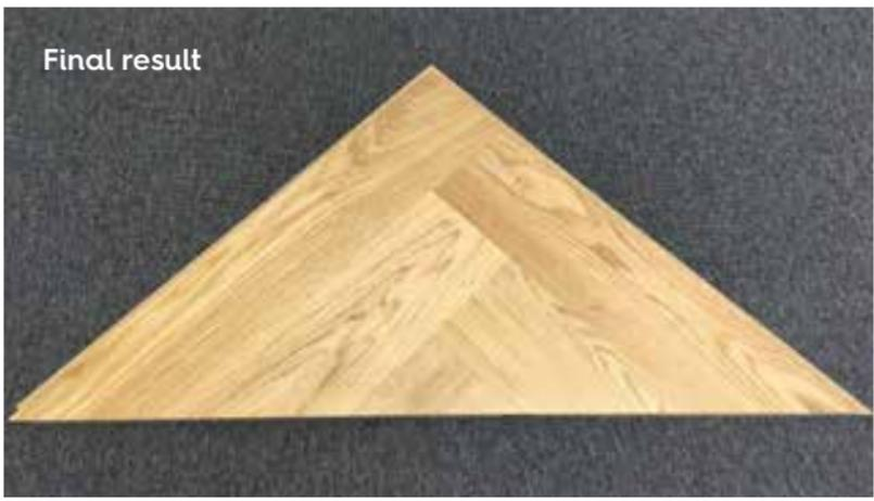
In case you have calculated and built an uneven number of triangles, leave the outer two triangles aside and lay out the middle triangles with their long side towards the starting wall.
